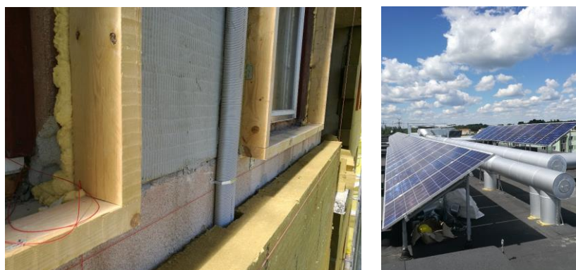
Figure 25. Ventilation pipelines in the external wall insulation, wooden frames to take windows in between the insulation layer (left) and PV panels (right).
